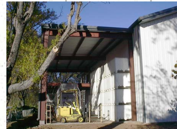
View of the "Crush Pad" from the South. The white boxes to the right of the forklift are our grape fermentors.
