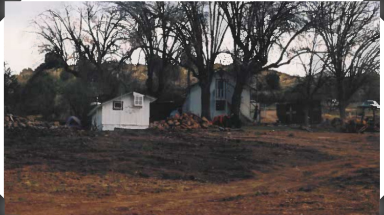
Two original buildings that still stand today – the Casita and Administrative Building.
