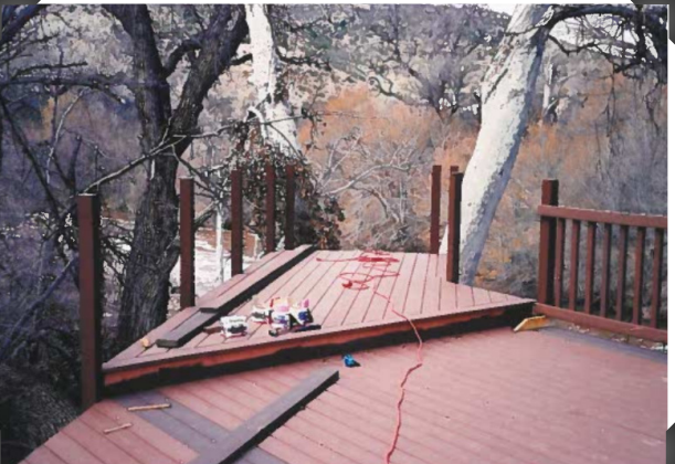
Creek Deck under construction.
