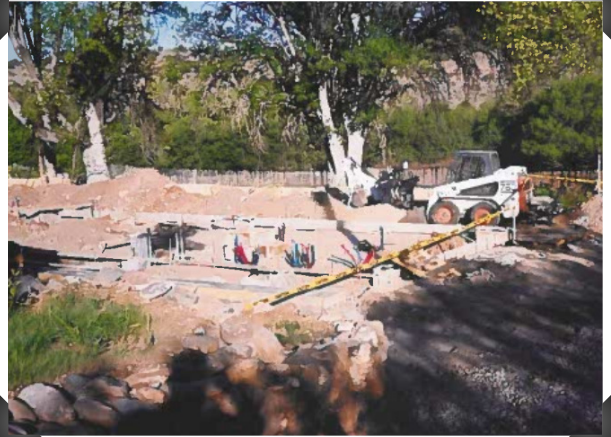
Beginnings of the Winery foundation.
